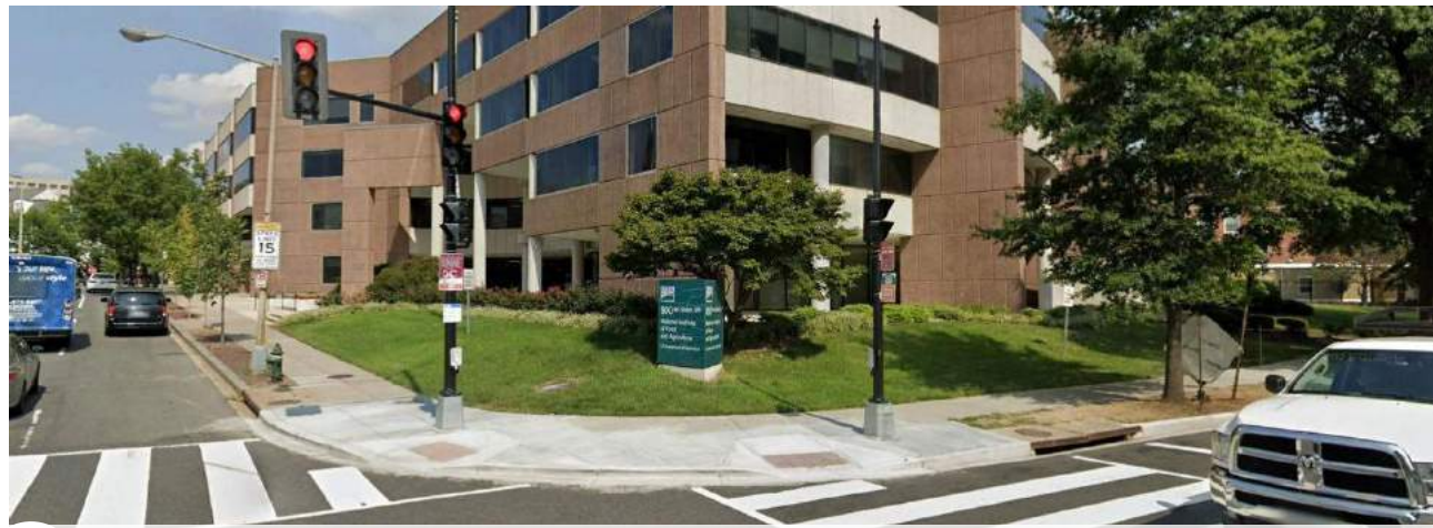
2 INTERSECTION OF 9TH STREET SW AND MAINE AVENUE SW
